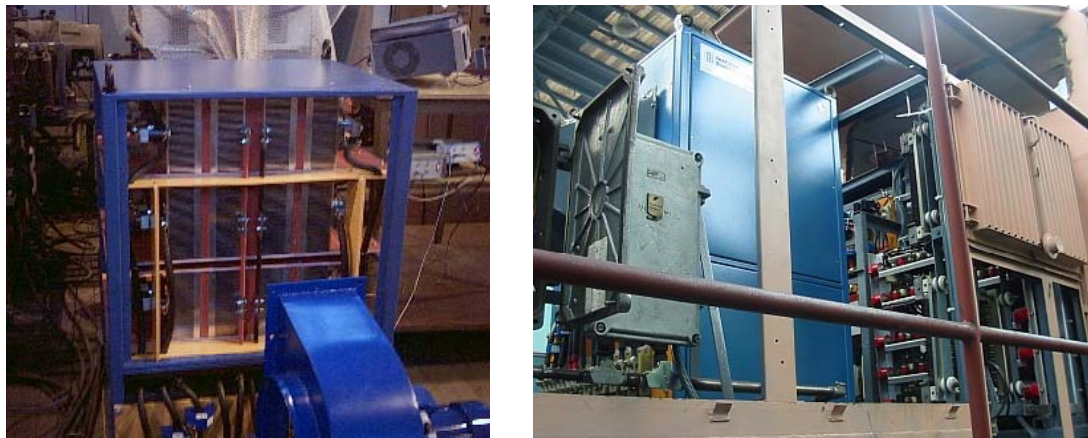
Figure 8: Refurbished chopper and installation
