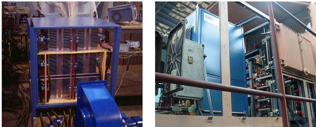
Figure 8: Refurbished chopper and installation
